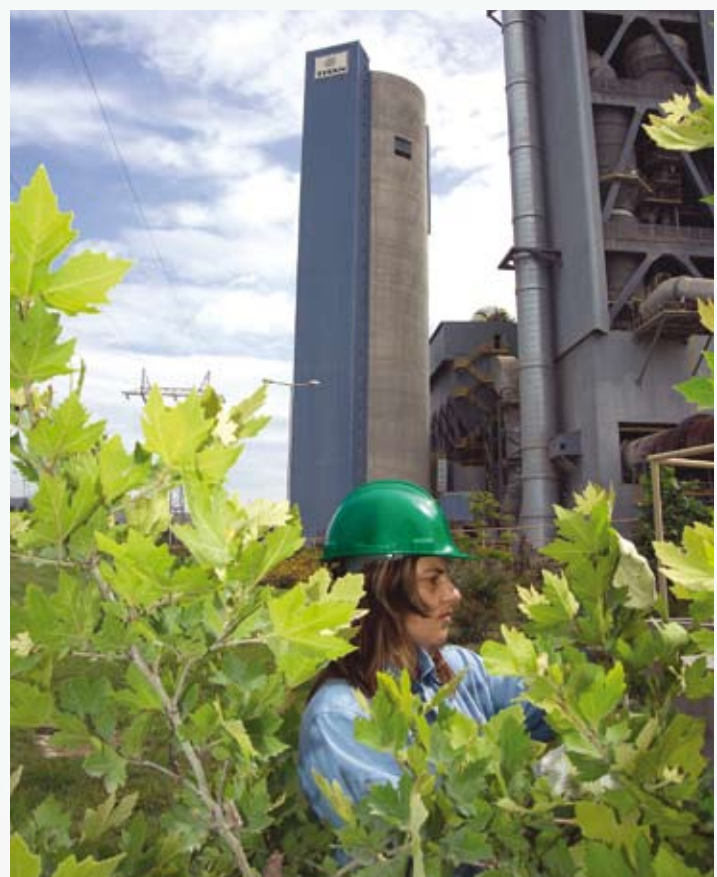
Thessaloniki plant, Greece
