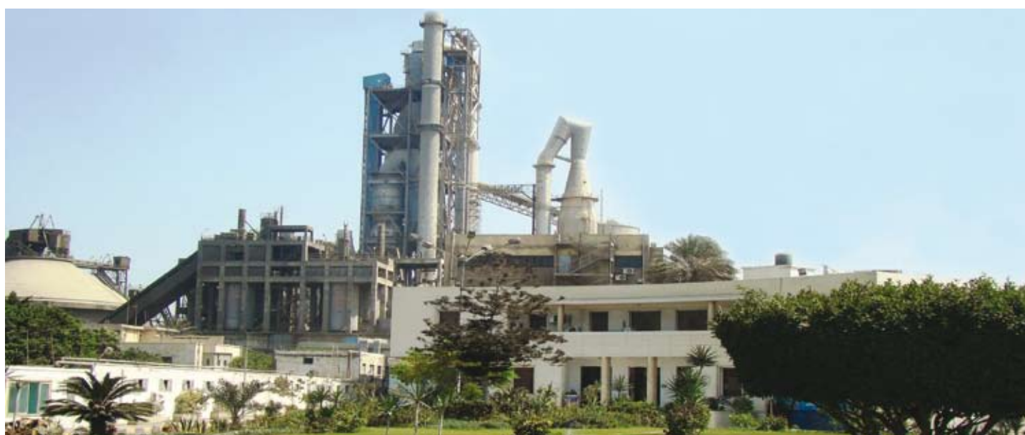
Alexandria plant, Egypt
