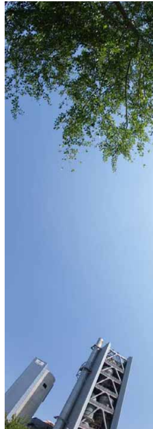
Thessaloniki cement plant, Greece
