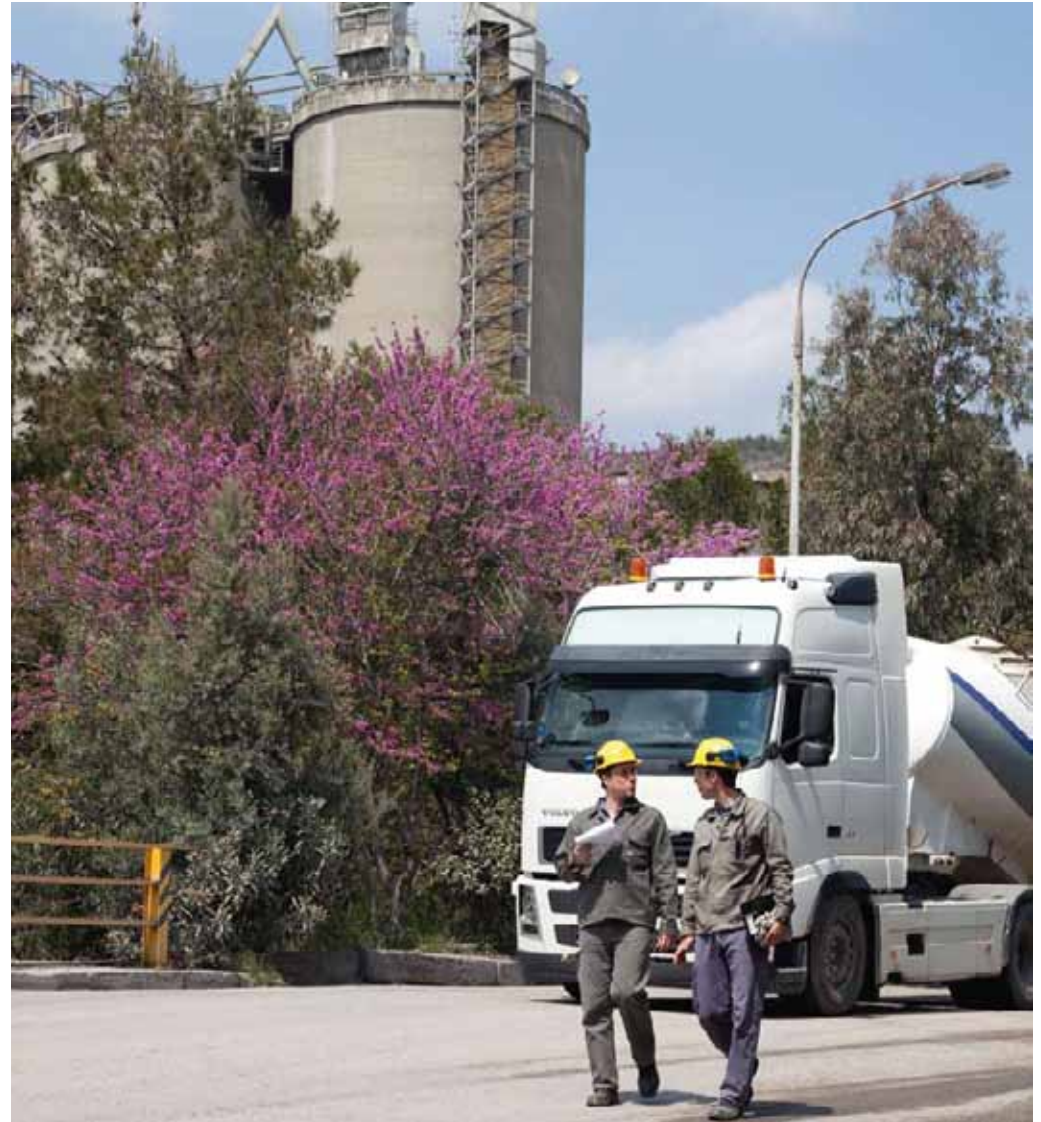
Kamari cement plant, Greece
