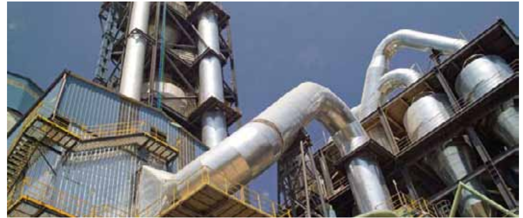
Antea cement plant, Albania
