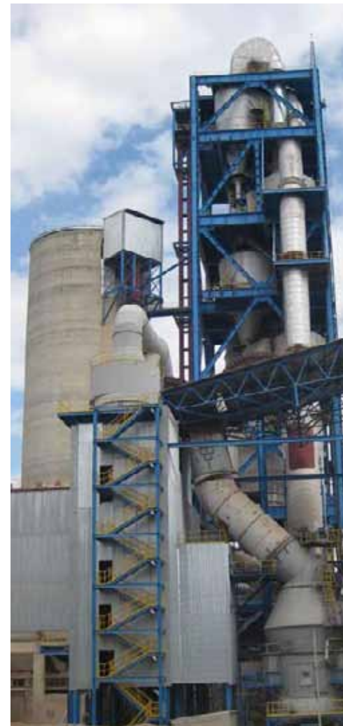
Adocim cement plant, Turkey
