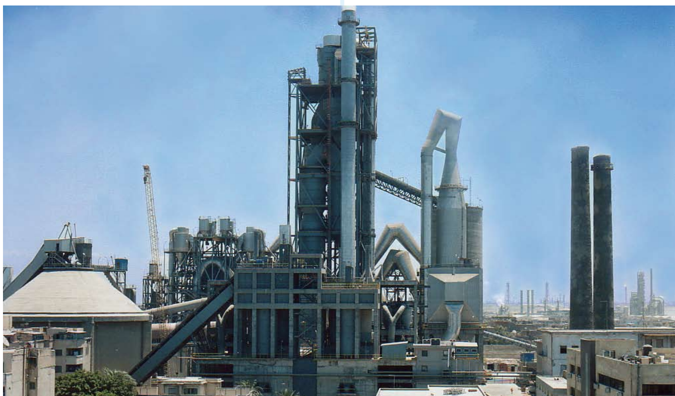
Alexandria plant, Egypt
