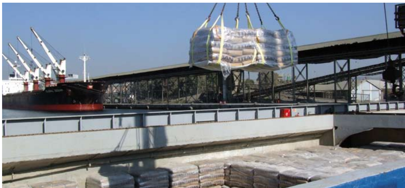
Elefsina plant, Greece
