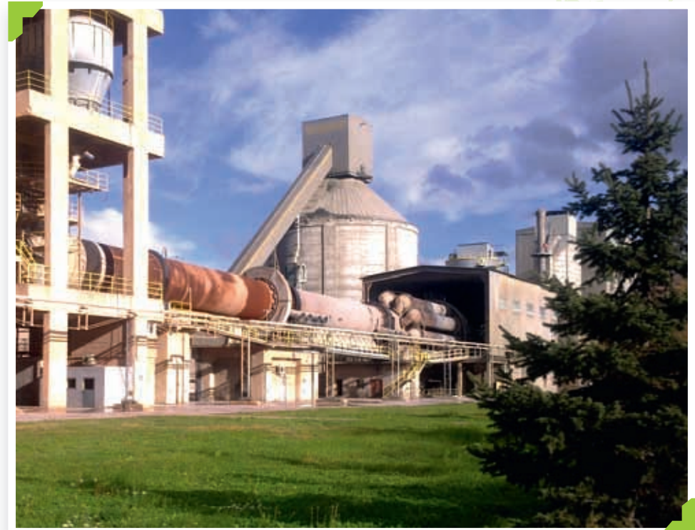
TITAN Kosjeric cement plant, Serbia
